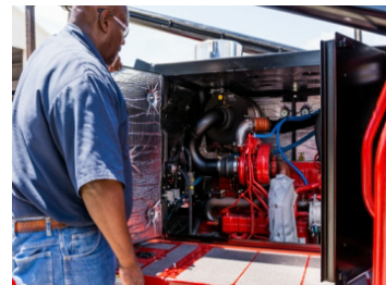
Service & Inspection from Ground Level
