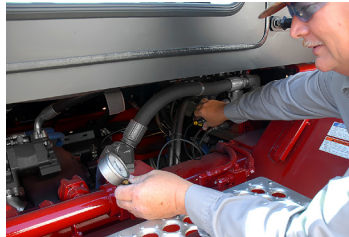
Service & Inspection from Ground Level
